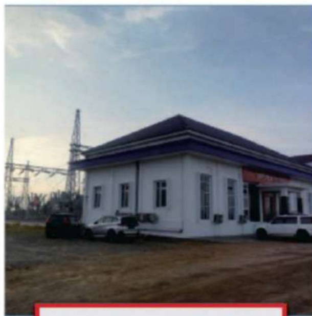
PT. NEW ASIA INTERNATIONAL GI 150kV 100 MVA
